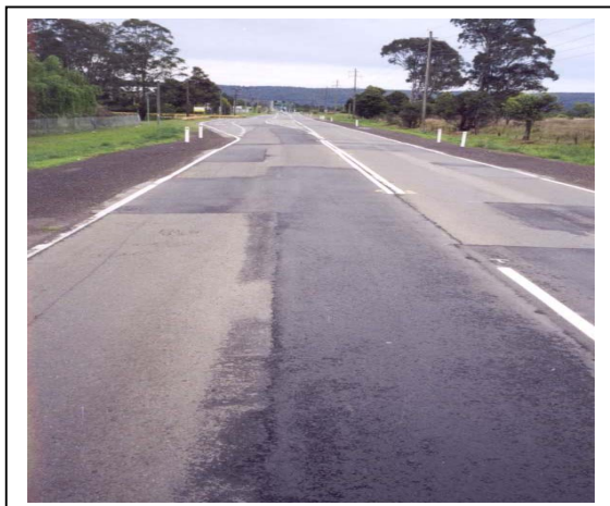
Figure 1.4.4 This section of road pavement has had approximately 20 – 30 % of the segment renewed.
