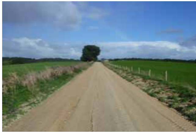
Partially completed resheet, final trimming and compaction delayed by rain, to be completed when material dries.
